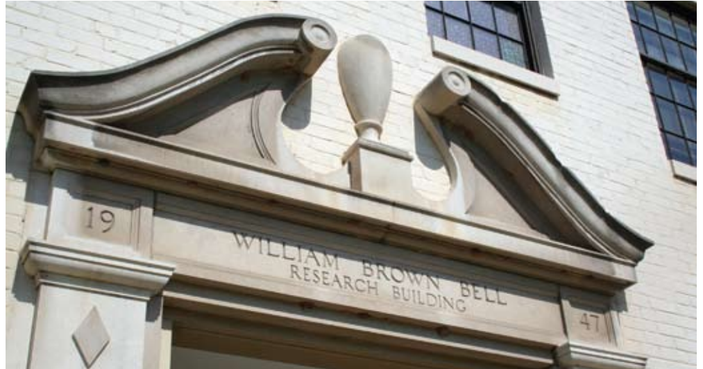
The historic Bell Building will be demolished in the Fall to make way for a new expansion to Duke University Hospital. Construction on the new building will begin in the Spring. PHOTO MARK SCHREINER
